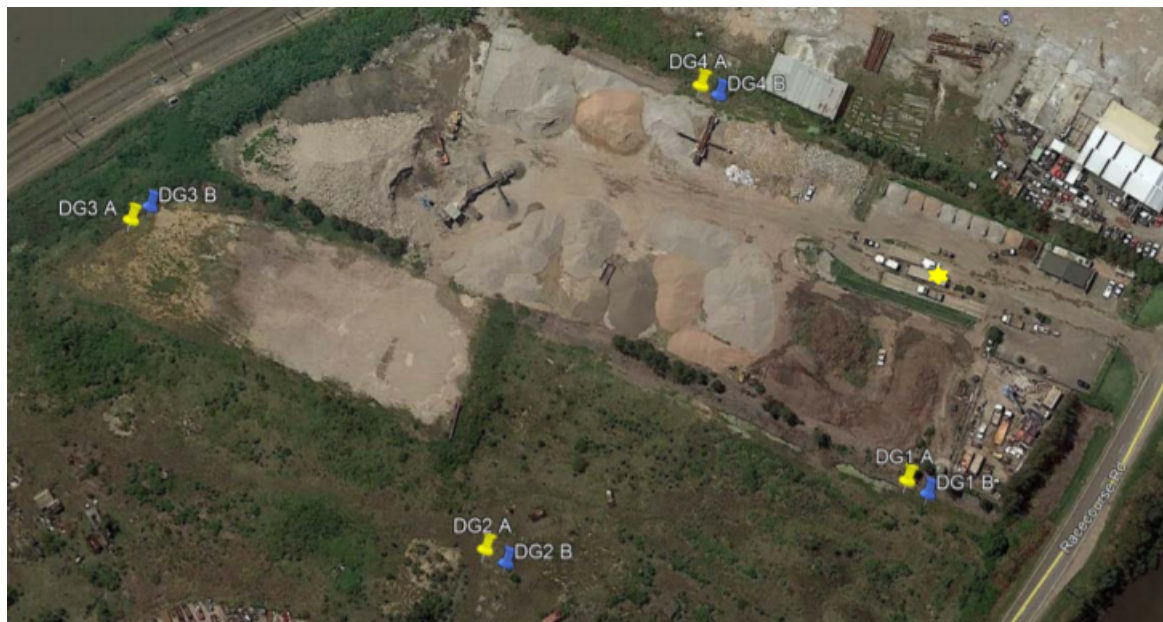
Figure 9: Concrush Facility - Dust Master and Depositional Bottle Locations
