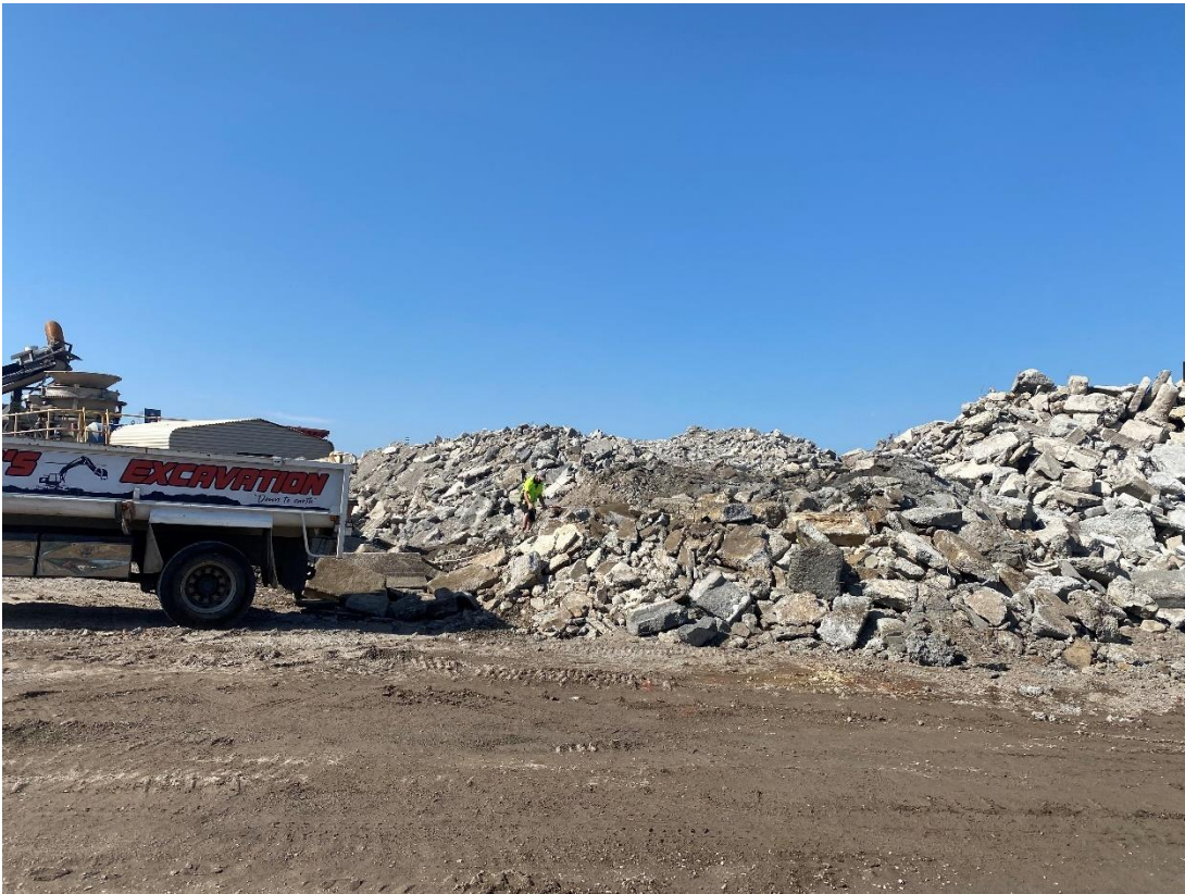
Photo 8 Concrete being loaded. No crushing on Day 1 of the site inspection.
