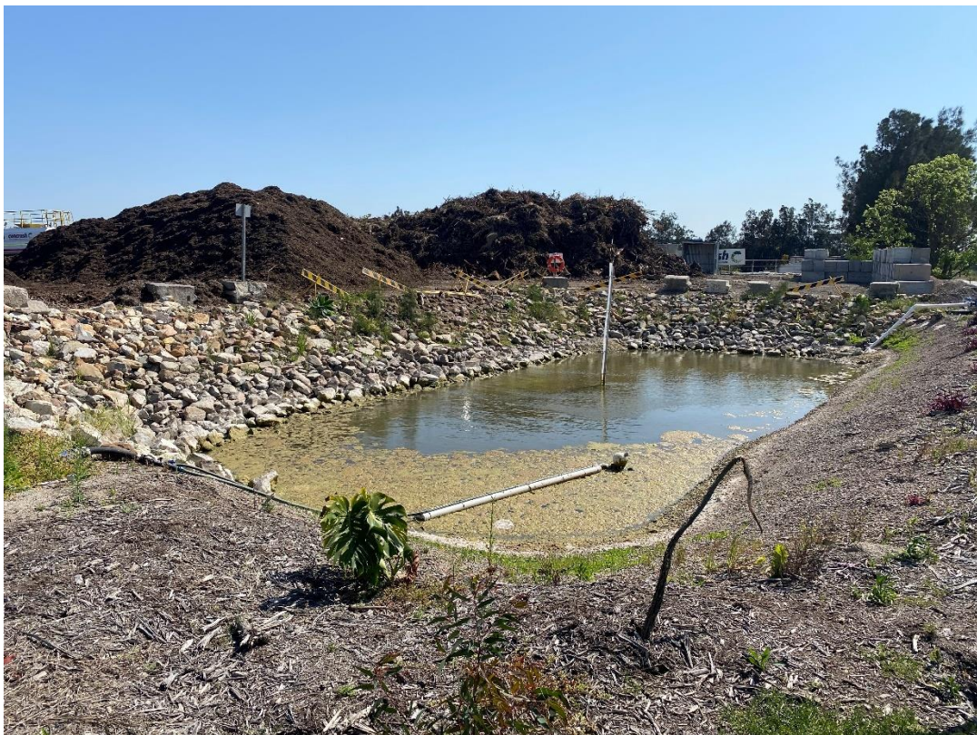
Photo 14 Leachate dam is stable.
