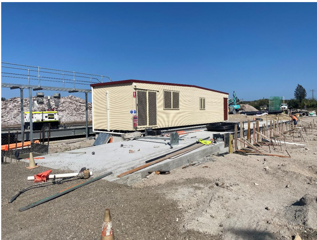
Photo 6 Stage 2 Operations weighbridge area under construction.
