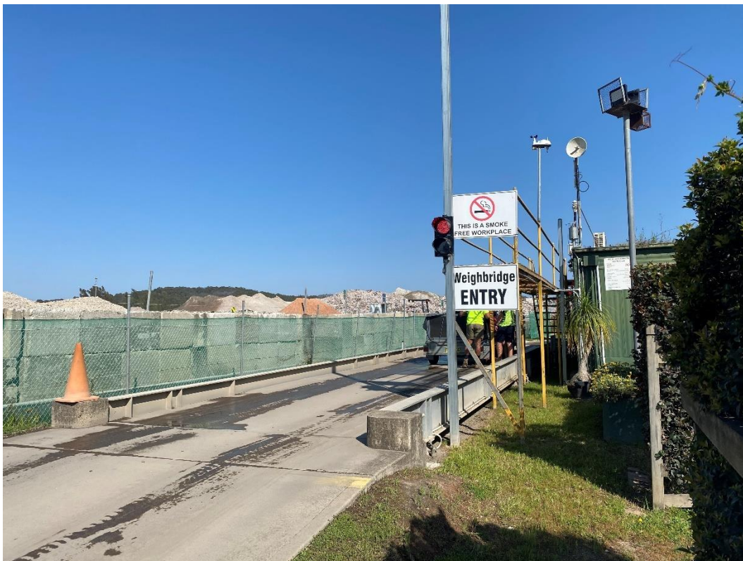
Photo 2 Weighbridge inspection for acceptance of material.
