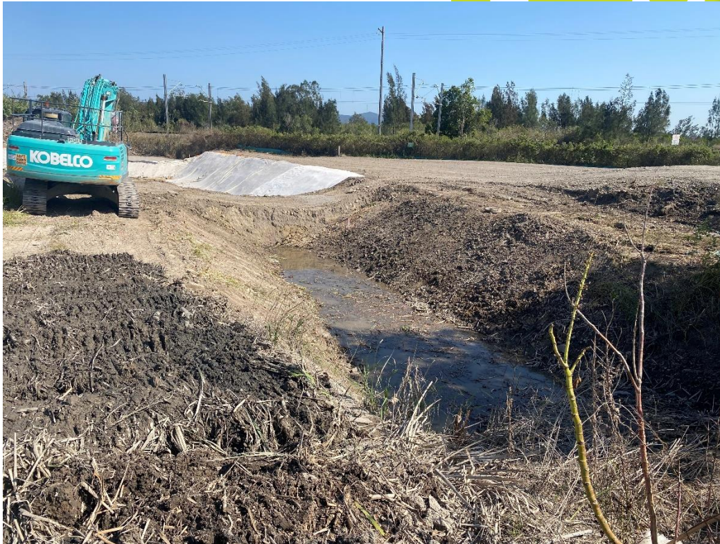
Photo 5 Sediment Dam 1 construction in the north-western corner of the site.
