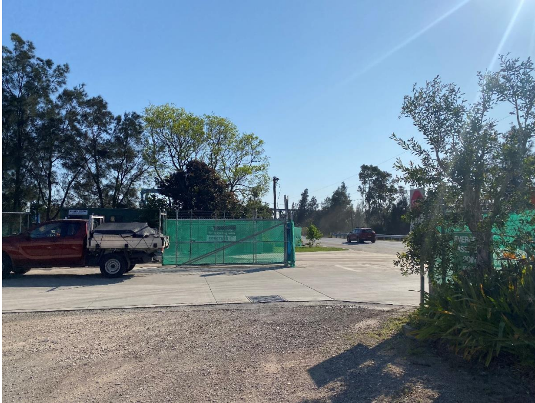
Photo 1 Clean entrance and intersection on Racecourse Road. Street sweeper and water cart in use during the site inspection.
