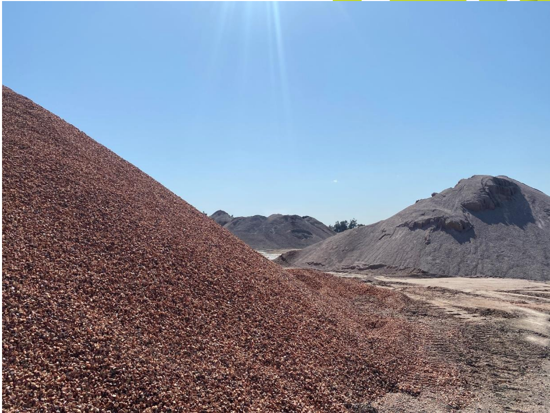
Photo 13 Crushed tiles and road base stockpiled in SSD Expansion area.
