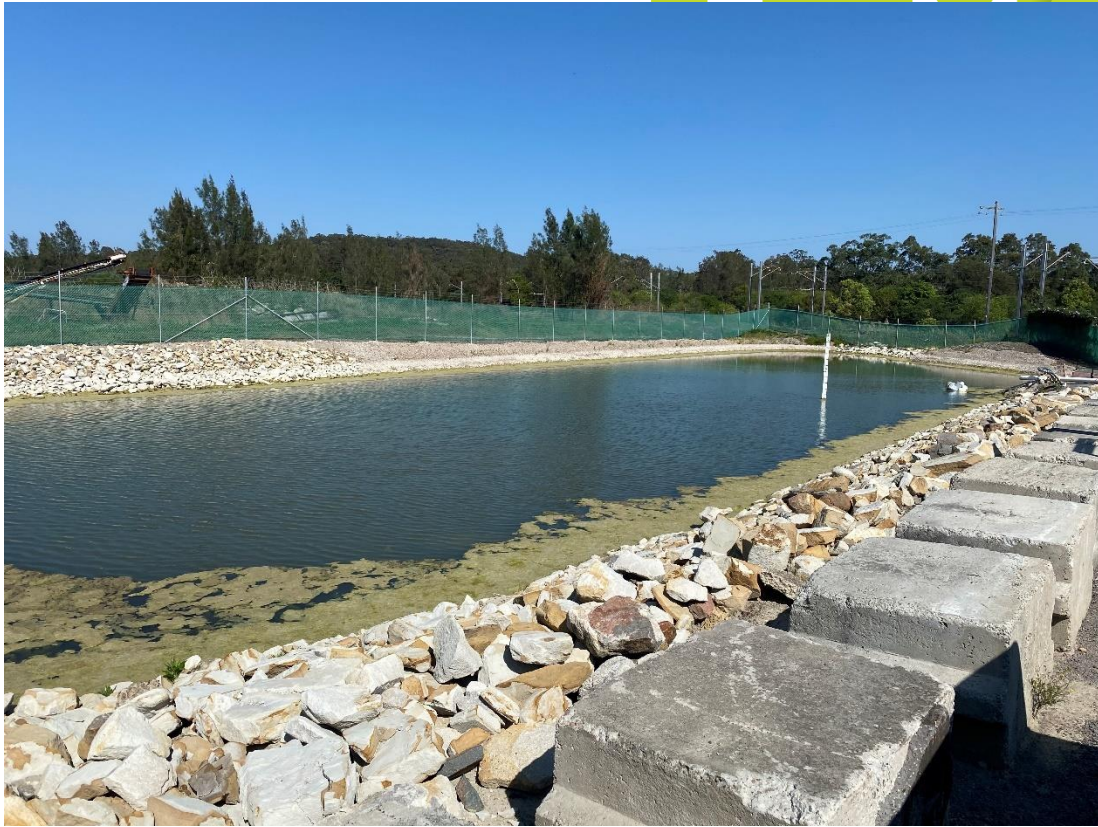
Photo 11 Sediment dam 2 is stable.
