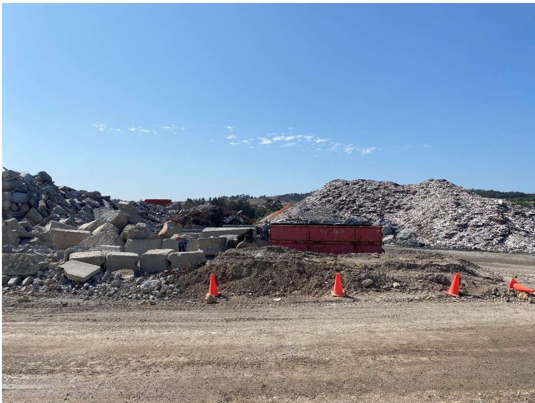
Photo 10 Boundary between SSD Expansion area and Council consent area.
