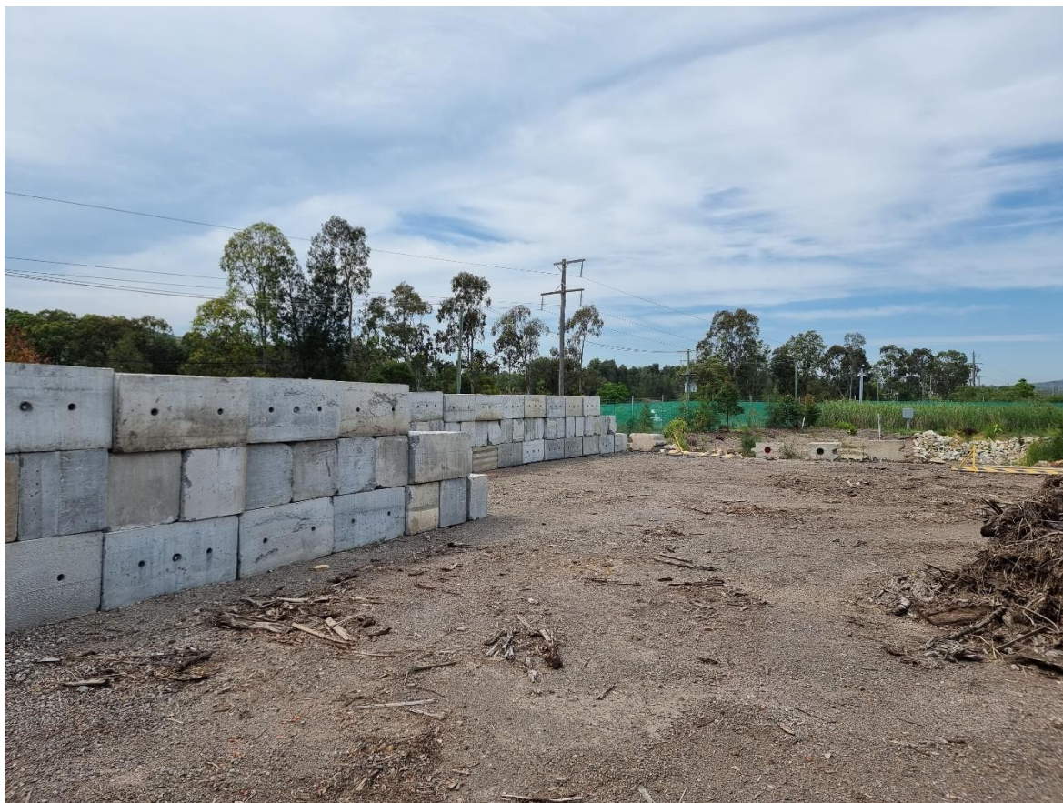
Figure 2 Green waste area noise wall under construction
