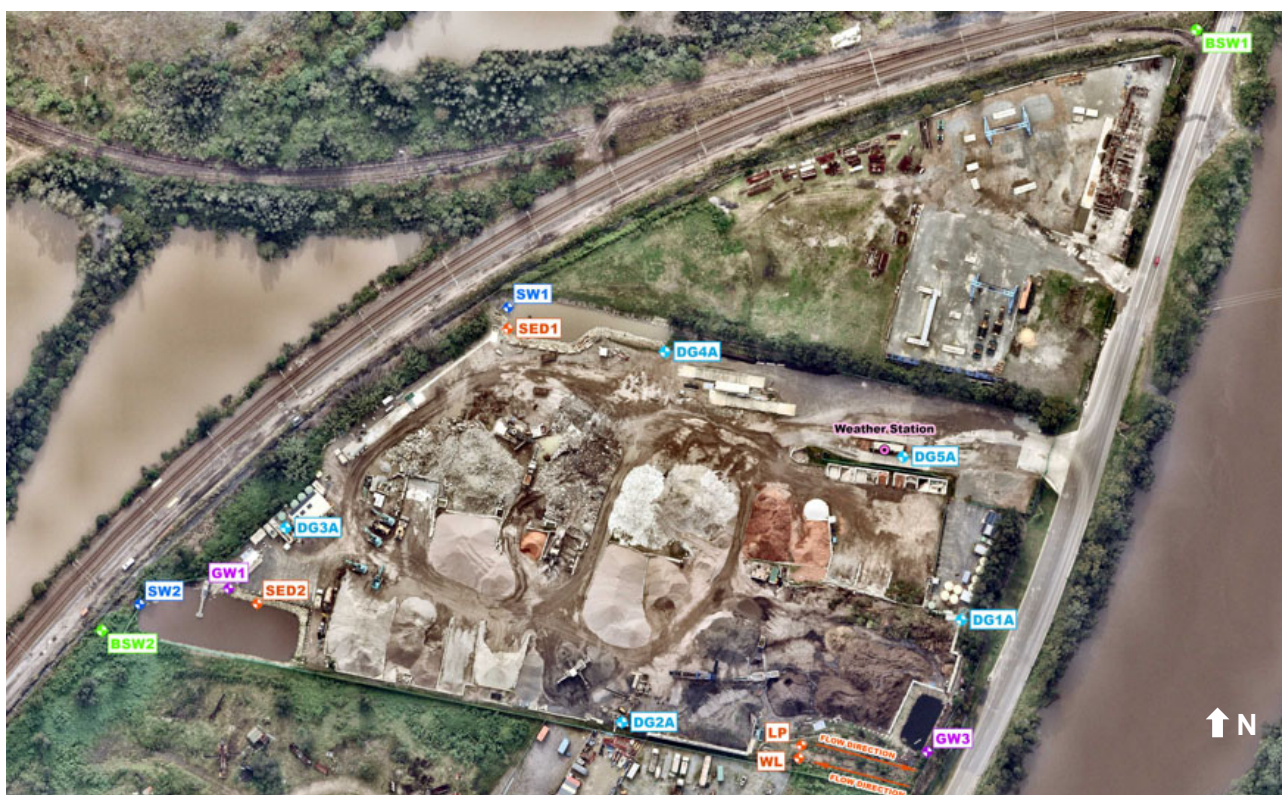
Figure 2 Water sampling locations (aerial as of 25 May 2025)
