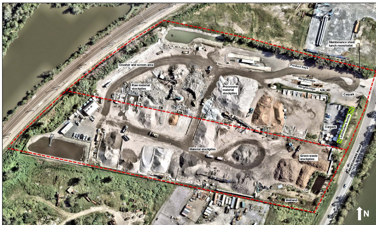
Figure 1 Project Site Location and Layout (aerial as of 7 February 2025)
