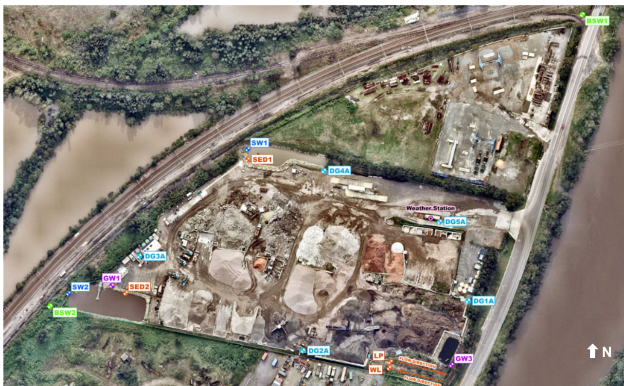
Figure 2 Water sampling locations (aerial as of 25 May 2025)
